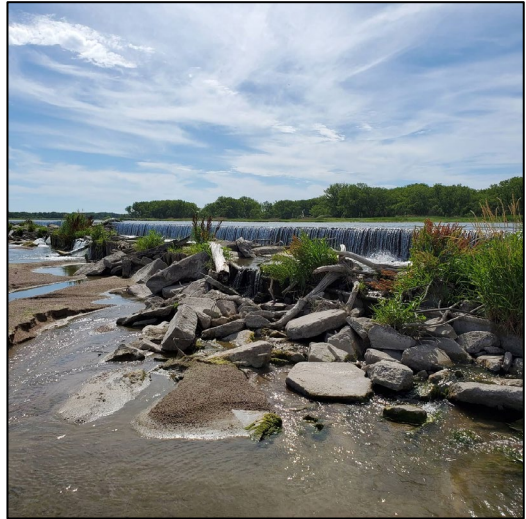
Water flowing over the Kearney diversion.
