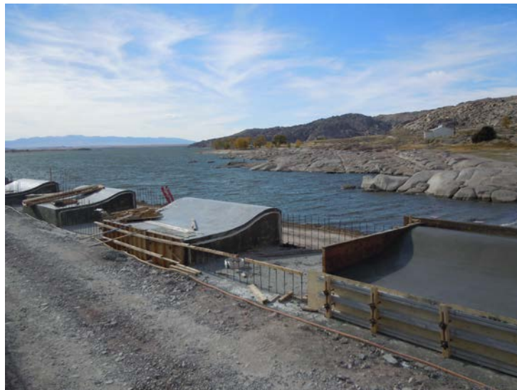
1881 Figure B-4. Pathfinder Dam ogee weir construction in 2011. 1882
